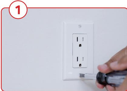
Carefully remove the existing screw from your chosen outlet cover. The screw will be on the bottom or the middle of the cover, depending on your outlet.
