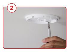
Using the 2 screws provided, attach the backplate to the desired location.
