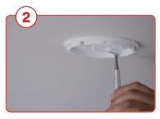
Using the 2 screws and a Phillips screwdriver, attach the base to the desired location.
