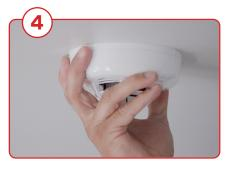
Take the detector and slowly twist it clockwise onto the backplate, until it clicks into place. There are markers on the backplate and detector to assist with alignment.
