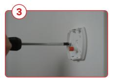
Secure the backplate against the surface, carefully filling in the two screw holes with the provided screws.
