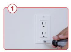
Carefully remove the existing screw from your chosen outlet cover. The screw will be on the bottom or the middle of the cover, depending on your outlet.
